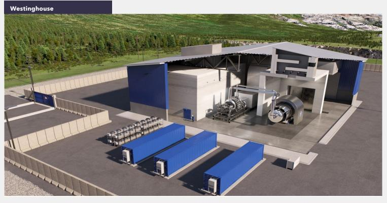
eVinci: The eVinci™ micoreactor from Westinghouse will be capable of producing 5MW of electricity for 8 or more years before refueling. The eVinci microreactor is air cooled and does not require water or pressurized gas for cooling. In late 2023, Westinghouse announced a partnership with the Saskachetwan Research Council to deploy the first Canadian eVinci microreactor, which is expected to begin operation by 2030.
